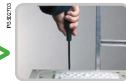
Make a small hole in the membrane.
